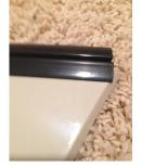
There should be a gap at the top of the panel to allow for the screw top. (Installed last)
